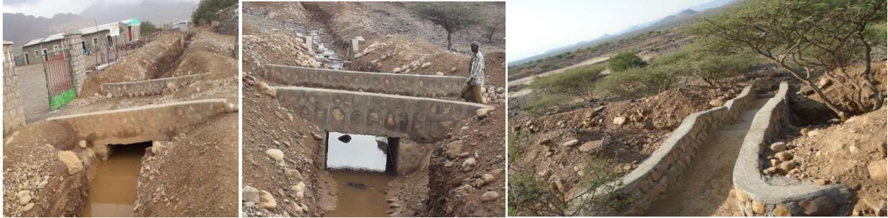
Figure 5: Road & Drainage culvert constructed
