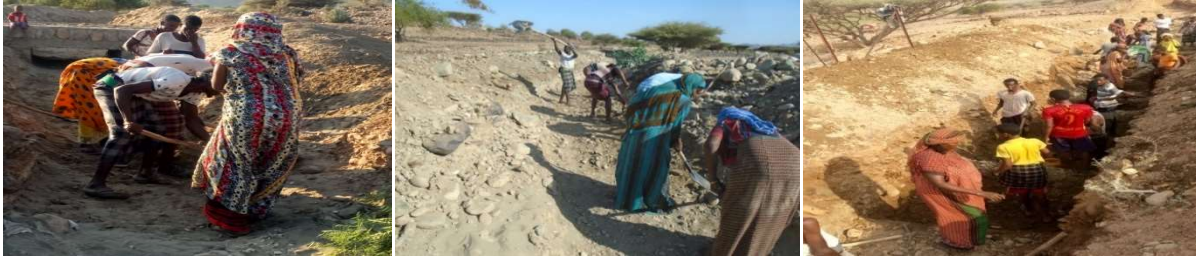
Figure 7: Main canal cleared from silt and debris
