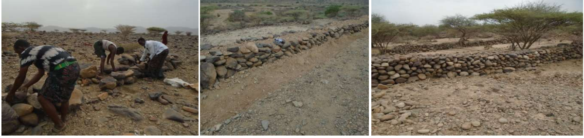
Figure 14: Stone check dams constructed
