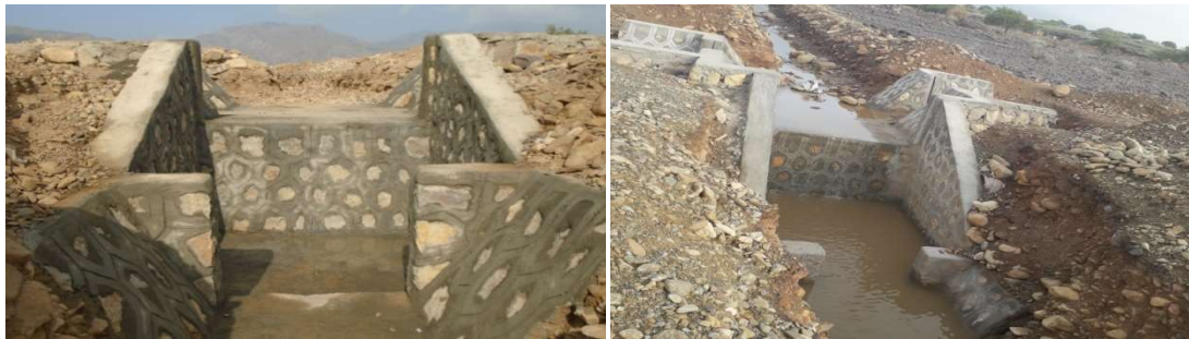
Figure 3: Drop structures constructed
