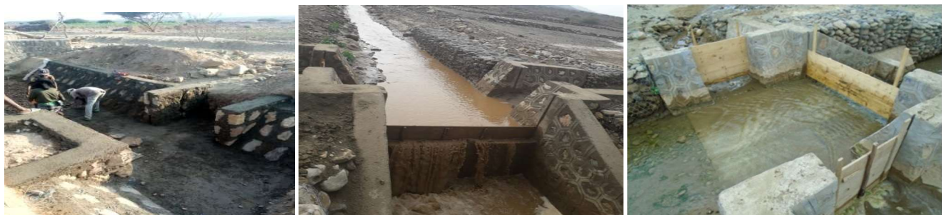
Figure 4: Division boxes constructed
