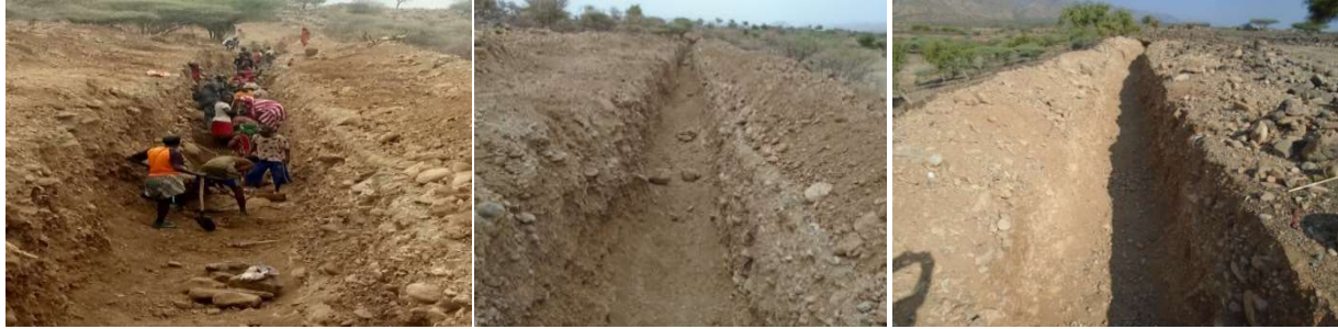
Figure 2: Secondary canal excavated
