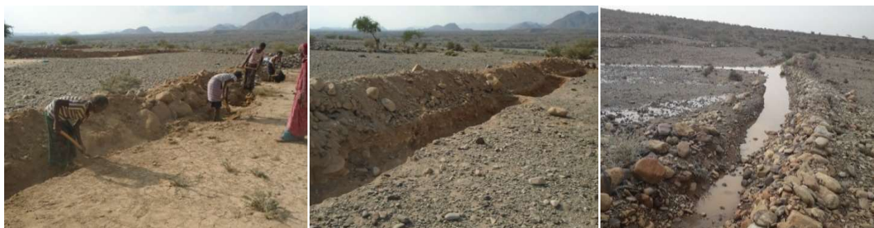
Figure 13: Soil & stone bunds constructed
