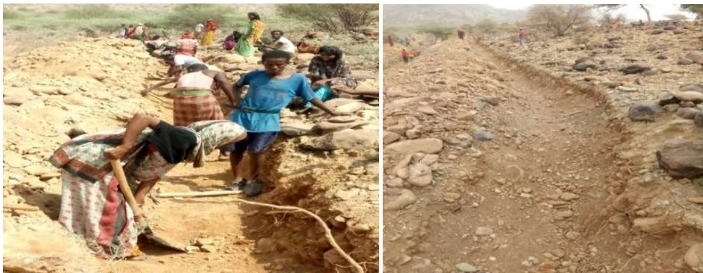
Figure 15: Cut off drain excavated
